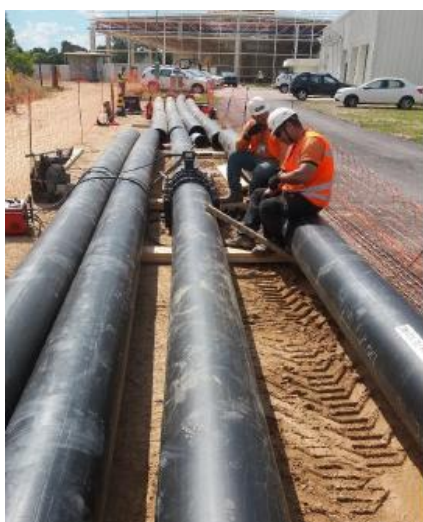
Solda dos tubos PE 100-RC FM APPROVED 355mm
